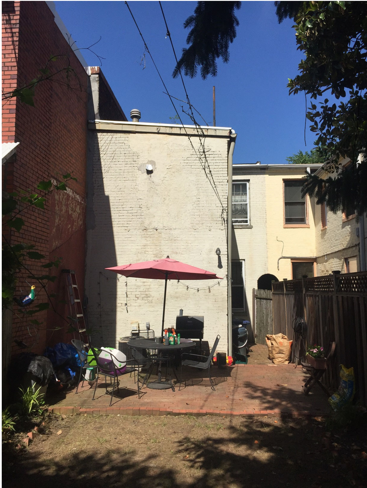
EXISTING REAR FAÇADE
