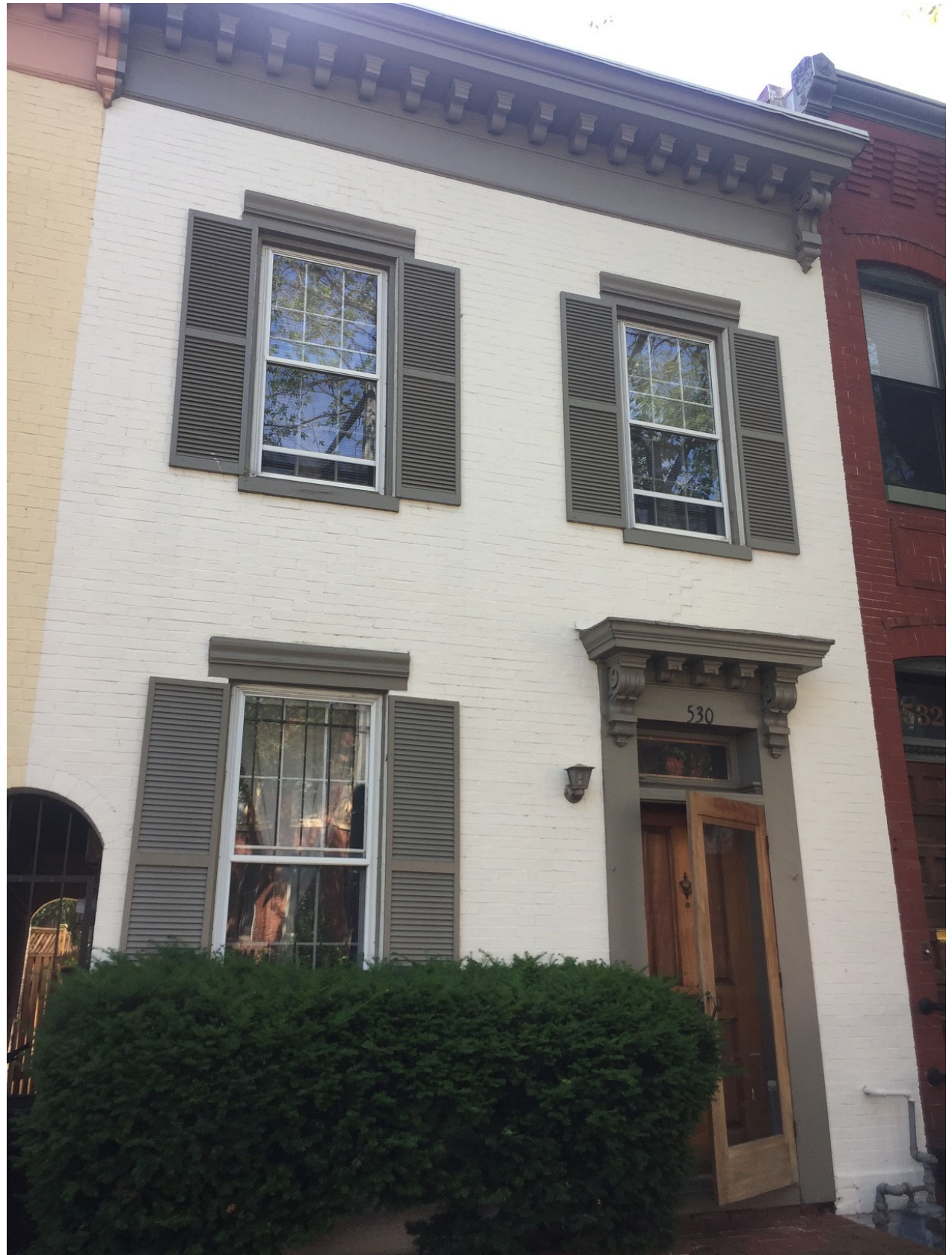
EXISTING FRONT FAÇADE
