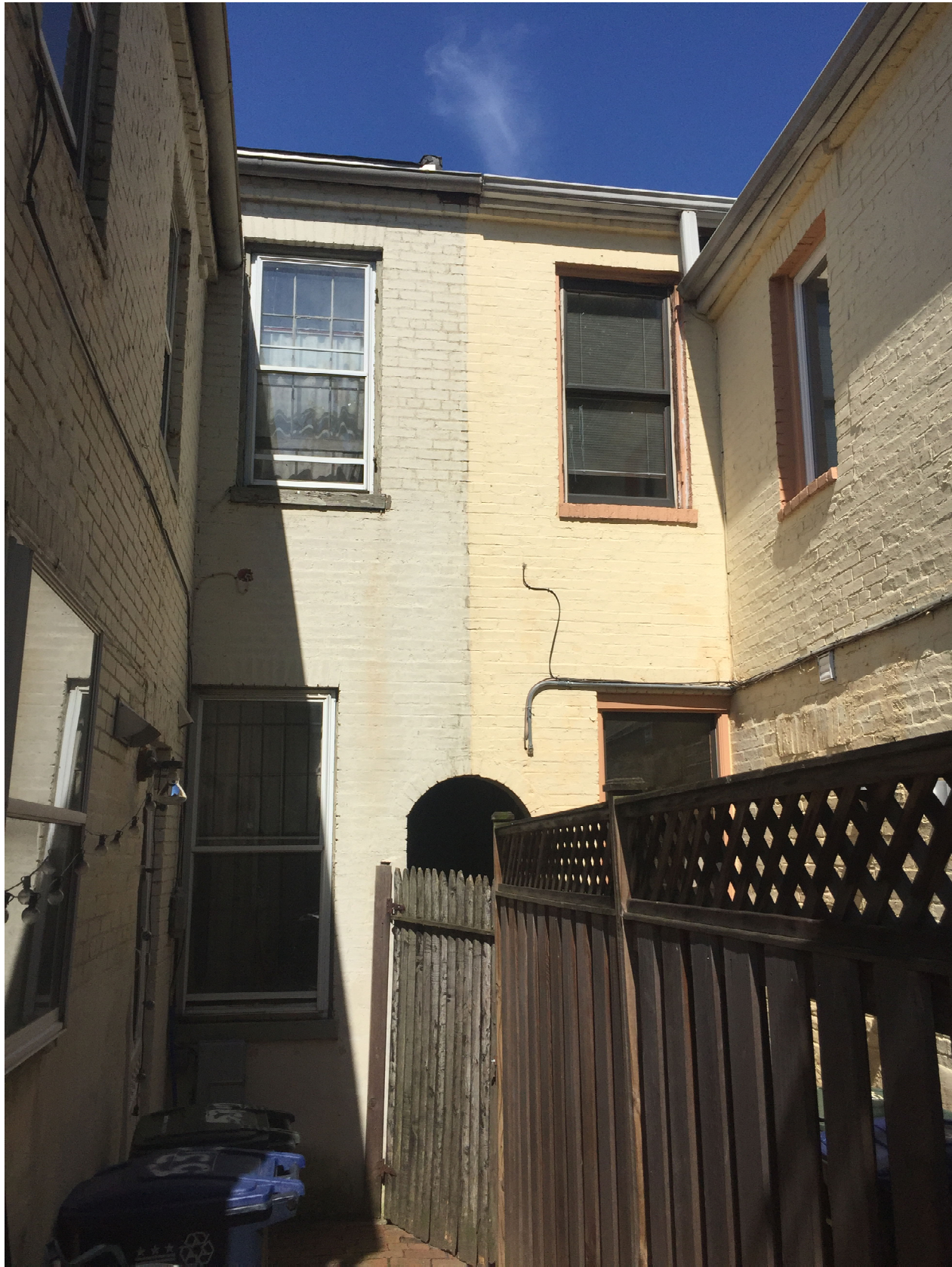
EXISTING REAR FAÇADE
